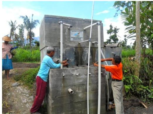
Gambar 5. Bak Reservoir dan Instalasi Pipa Distribusi
