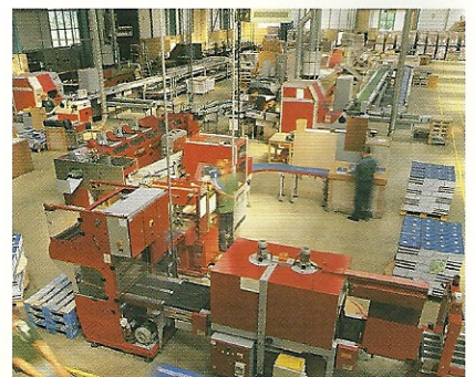
Example of conveyor belt control.
