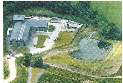
Example of remote pumping station.
